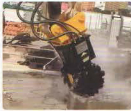
建筑物拆除 building demolition
